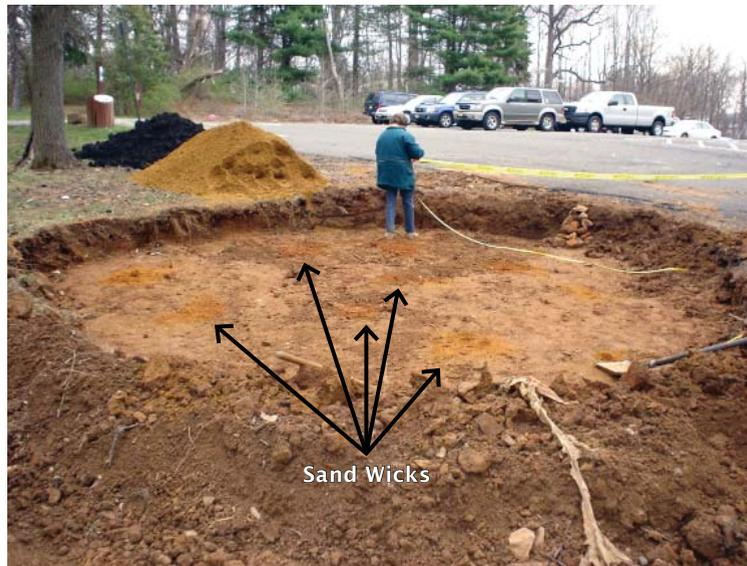
As illustrated in the image on the left, in addition to the recommended soil amendments, it may be helpful to add sand wicks to a rain garden site with clay soils. To do this, dig out holes, preferably 1 foot deep if possible, and fill in with pockets of coarse sand. This will increase the infiltration capacity of the rain garden.
